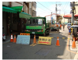
(j)漏水點開挖前
