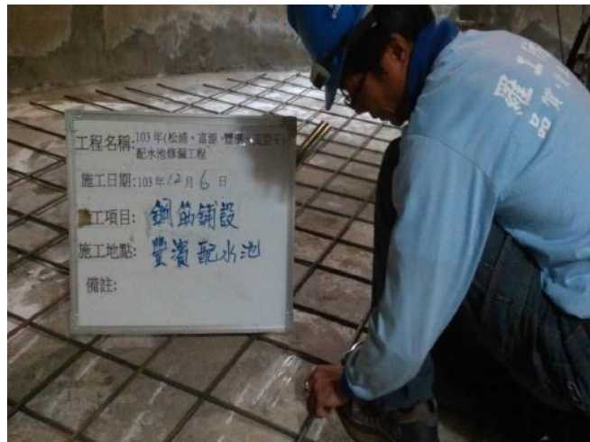
6.池底鋼筋綁紮
