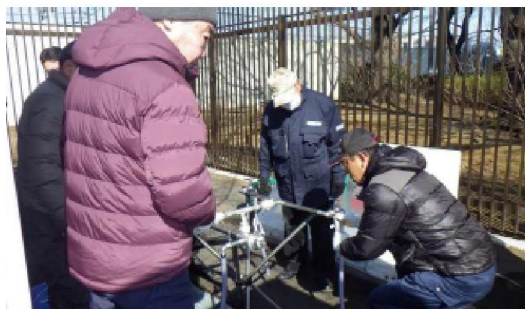
Experience of setting up temporary hydrants
