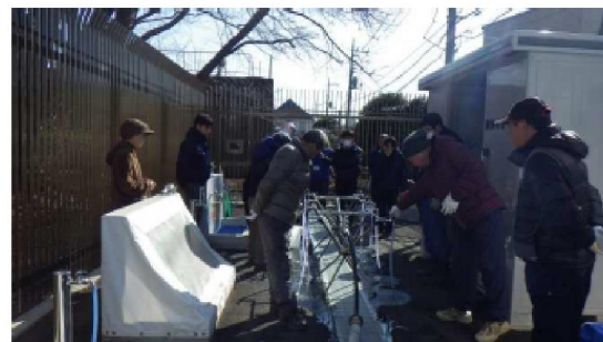
Checking of water flow
