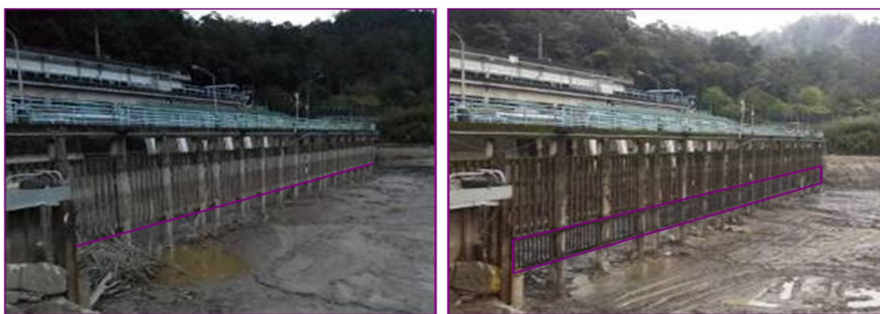
隔欄柵施工前
