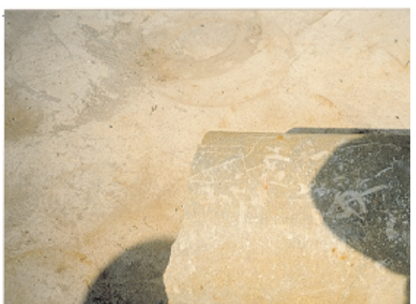
員林鎮山腳路3段3號前350mmACP斷裂
