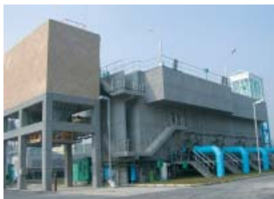
澄清湖淨水場新設結晶軟化池 Pellet Softening Reactor
