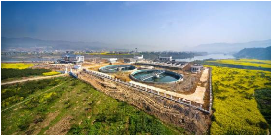
Beijing Capital's Yangjiaxi Wastewater Treatment Plant
