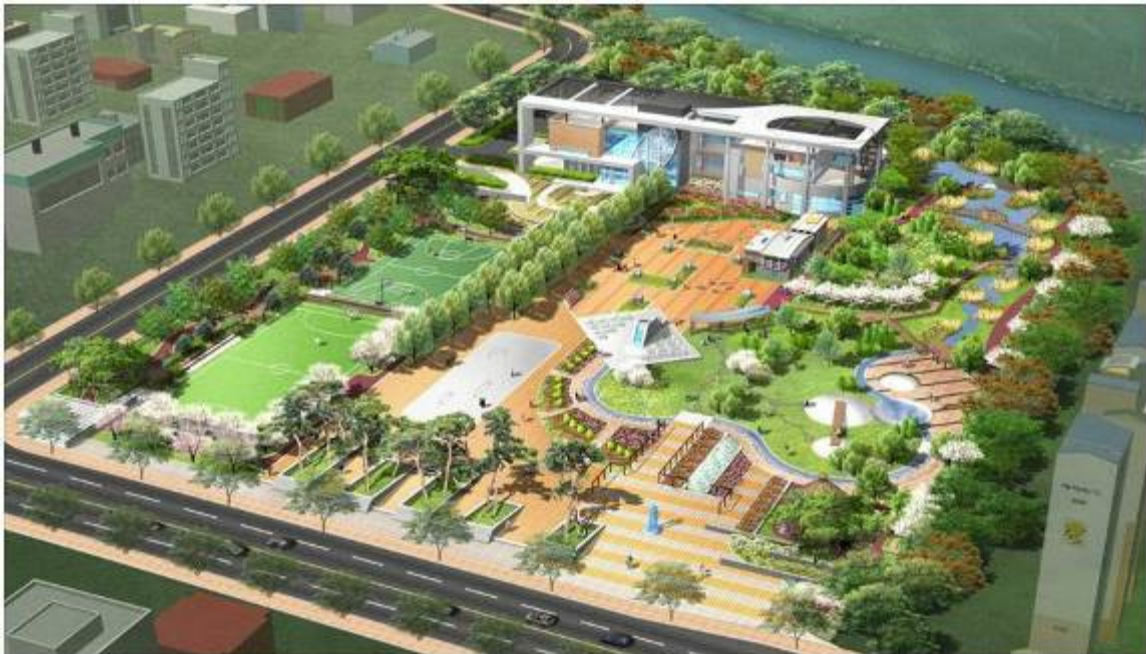
Aerial view of the YongIn YoungDuk Sewage Treatment Plant.
