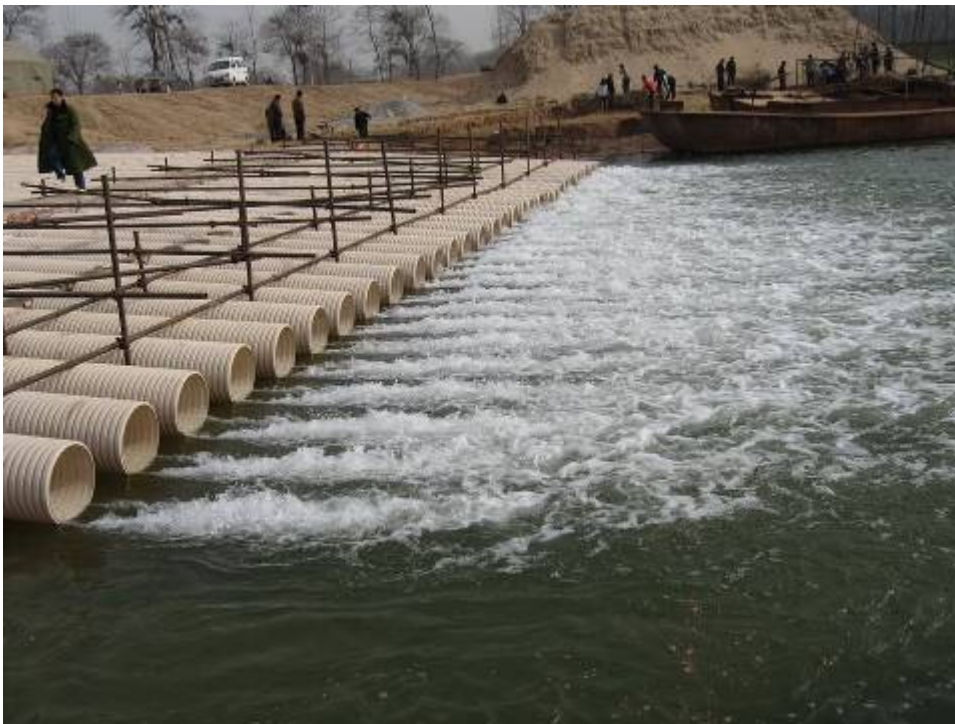
Remediation of Dasha River to meet downstream requirements.
